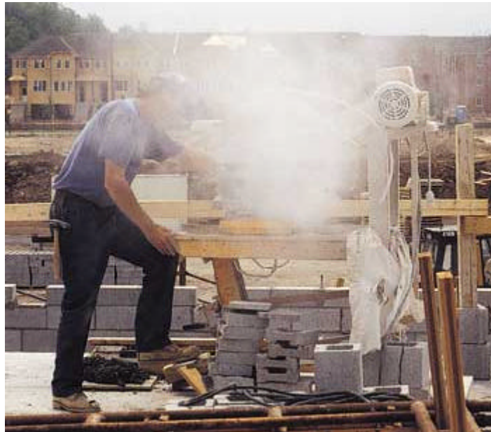
Dry cutting generates high levels of dust
