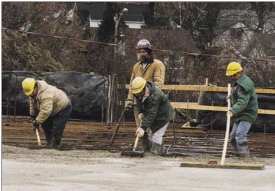
Waterproof rubber boots are essential in working with wet concrete
